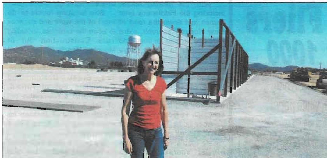
Donna Martin Whitaker is the owner of the new storage facility being built in the Toyon area. Units in the first phase of construction are expected to be available in a month.
